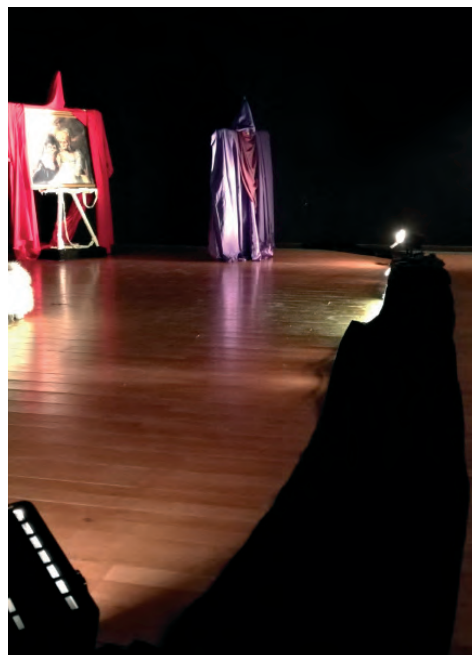
Photos showing the black fire proof cloth covering the cables/halogen spots.
